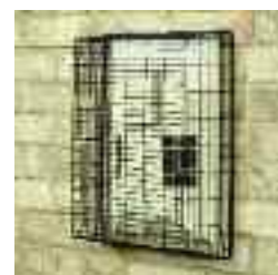
Recessed rear vent terminal (for use if external space is restricted)
